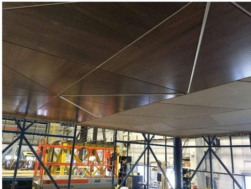
**Figure 2 - Custom cross tee lights (system 18B)**
